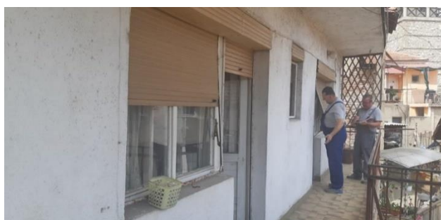
Figure 2 - Reconstruction of a housing unit in Veles in progress
